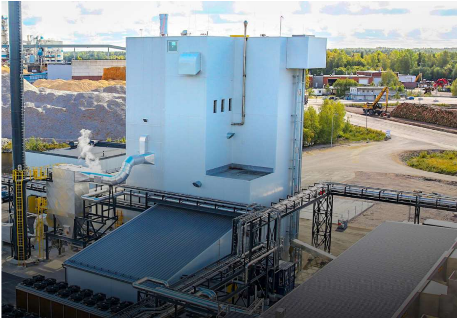
Figure 2: BTG pyrolysis plant in Gävle, Sweden, with capacity 40 000 tons of biomass per year. Source: https://www.btg-bioliquids.com/plant/pyrocell-gavle-sweden/
